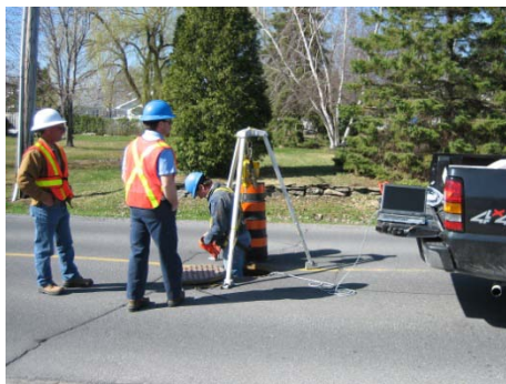
Manhole Location Selected for Flow Survey
