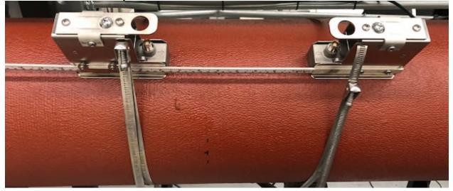
6. If you need to make fine adjustments  $(\pm 0.25")$  to the spacing at this point, you may do so by loosening the hose clamps slightly, and sliding the brackets while the transducers are installed inside them. Tighten hose clamps when done.
