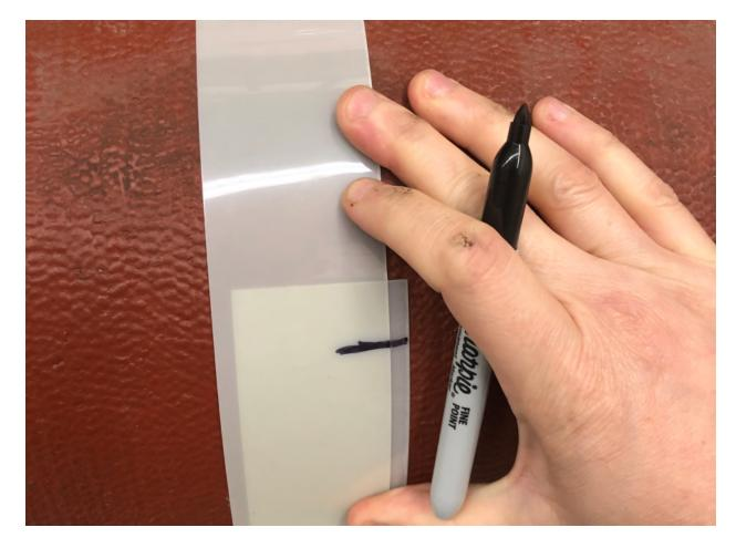
7. Lay the mylar sleeve flat, use duct tape to help hold it flat if you need to, and use the tape measure to measure half way between the two marks created when you wrapped the mylar around the pipe:
